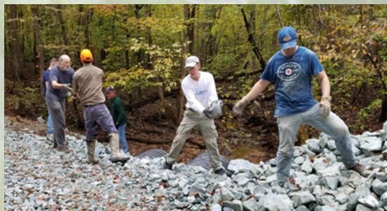
Volunteers help repair a culvert washed out by Hurricane Florence.
