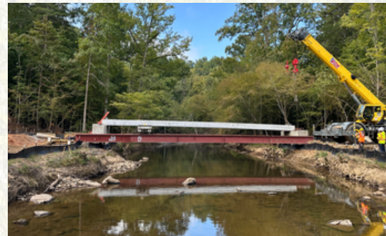
The new, clear-span bridge has taken shape! The foundational concrete pillars and slabs are in place and work to create the deck surface and install railings is ongoing.
