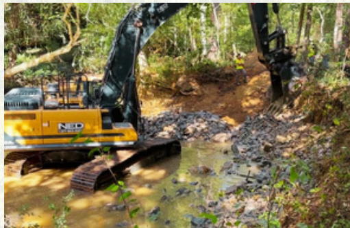
The materials from the demolition of the Billy Erwin Dam have been repositioned to help stabilize the highly eroded streambanks nearby.
